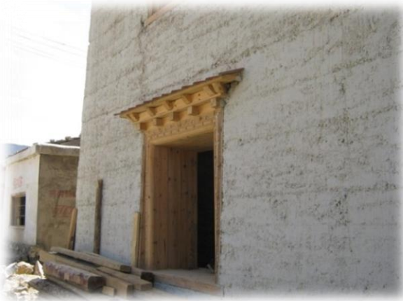
A three storey building in China - note lines of raised shuttering
