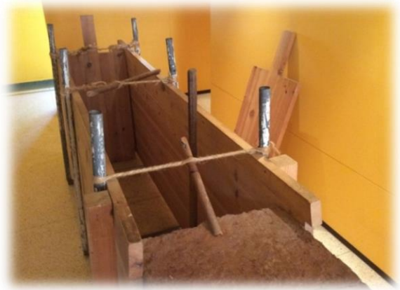
Shuttering for a rammed earth wall in Morocco
