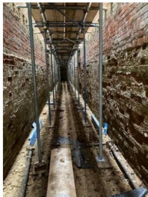
Interior scaffolding in place whilst the new frame and roof are installed.
