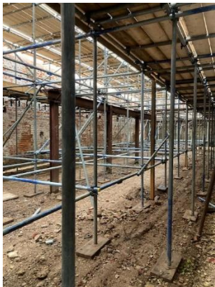
Interior scaffolding in place whilst the new frame and roof are installed.
